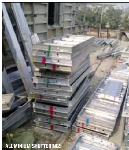
ALUMINIUM SHUTTERINGS Deshuttering of the panels
