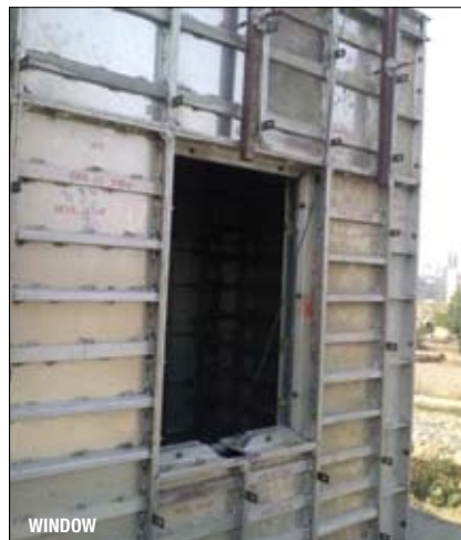
WINDOW Wall panels fixed with pins
